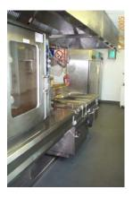
Due to the existing equipment type and construction it was not possible to simply replace individual elements i.e. replace the defunct oven and as it was proving very difficult to find a repair route, replacement of the suite seemed the practical solution.
