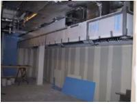
Being a new build there were areas of overlap between the construction and fit out as items such as cold rooms and ventilation canopies etc. needed to be installed within the construction phase to enable follow on services and construction works to be completed.
